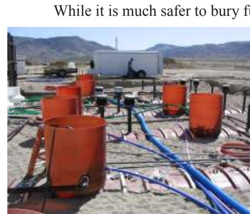
While it is much safer to bury fuel tanks, it makes any leak difficult to detect. Prior to the UST rules, a gasoline leak of a few gallons a month was cheaper to ignore than to fix. However, small leaks accumulate leaving a plume of fuel in the ground below.
